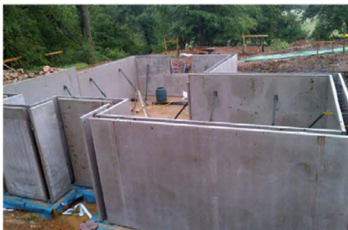
Double wall installation
